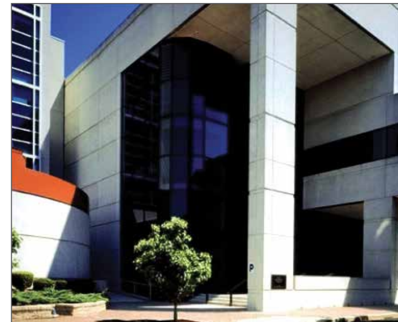
Vetter dedicates its first facility located outside Germany.
