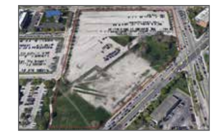
The IMD Gateway development, estimated to open in 2016, will include retail and lab space, a hotel and medical offices.
